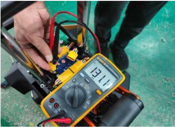
16 Full battery voltage check
